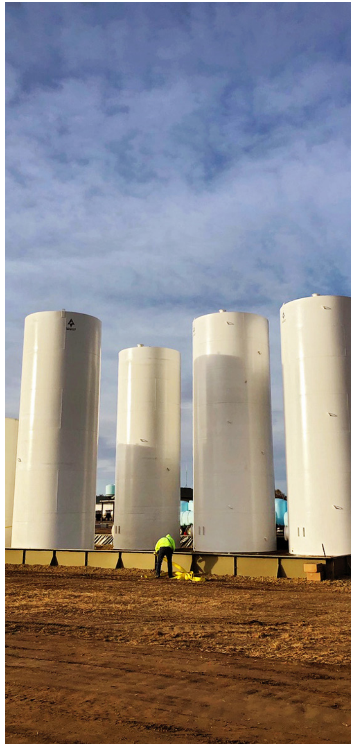
Construction of a new energy bulk plant at the Central Valley Ag location between Long Pine and Ainsworth, Nebraska. This new bulk plant will feature eight upright tanks with 215,000 gallons of diesel and gasoline capacity. It will allow consolidation of three current bulk locations each of which needed safety and environmental upgrading.
