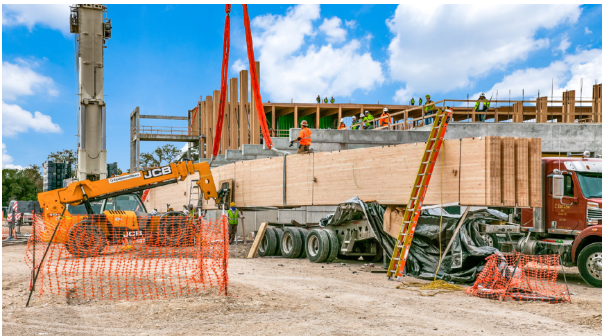
L: Prepping to place the 130-foot glulams into place via crane in Nov. 2022. R: Employees Alex Arrunada and Brad Longe admire the facility during a site visit on Jan. 23, 2023.
